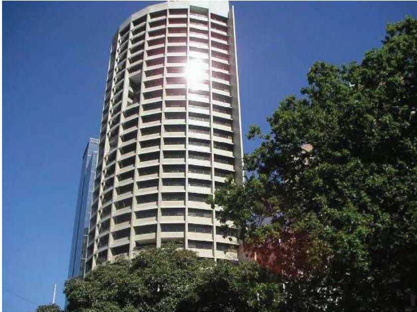
**Figure 10.** Precast concrete structural facade elements at Shell House in Melbourne, Australia.
