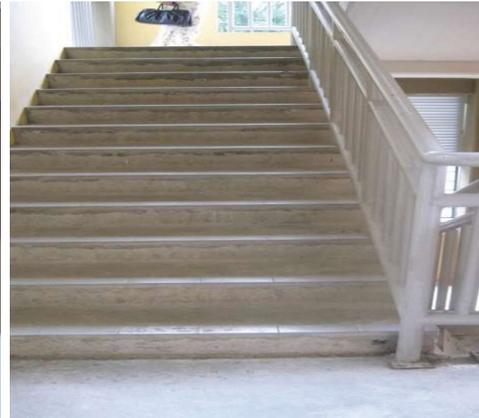
**Figure 4.** Consistent height of staircase riser (IBS Method)
