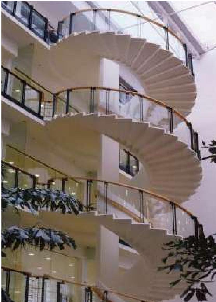
**Figure 6.** High strength concrete with a compressive strength of  $250 \text{ N/mm}^2$  used by Alborg Cement in Denmark to construct this precast concrete spiral staircase. c. Alborg Cement.
