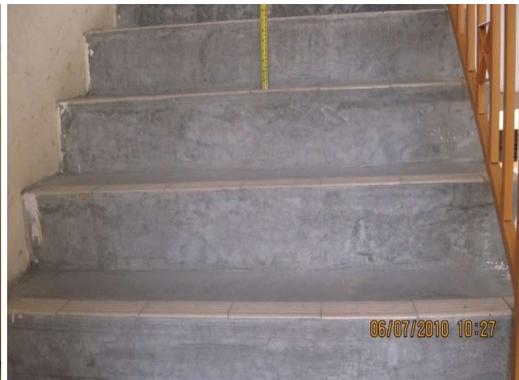
**Figure 2.** Inconsistent height of staircase riser (Conventional Method)
