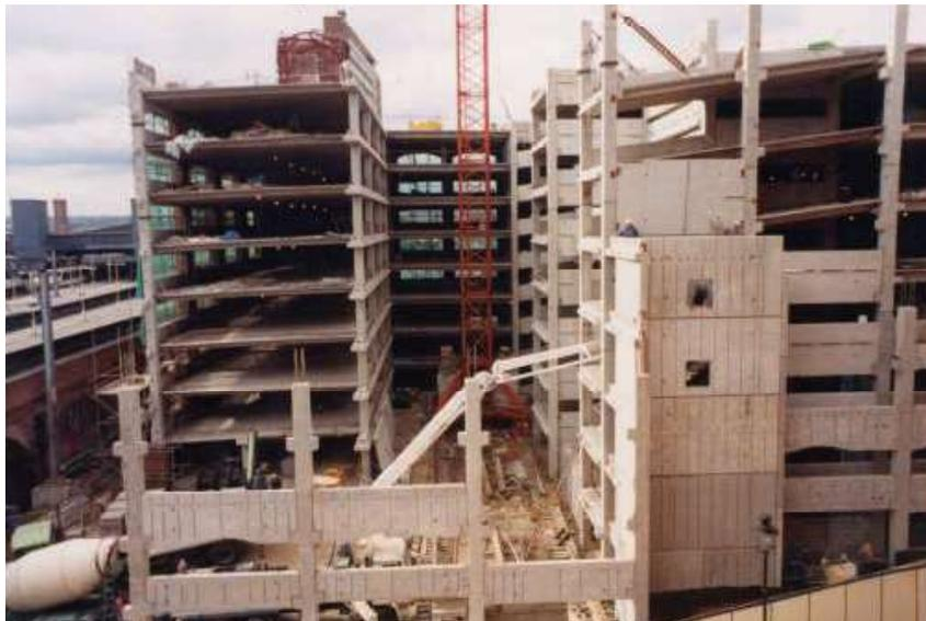
**Figure 3.** This shopping centre and car park uses a wide range of precast concrete elements. This is a so called skeletal frame, comprising beams, columns and slabs, using concrete shear-walls for stability.
