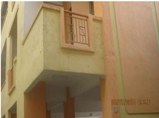
**Figure 1.** Poor plastering finishes of wall and column (Conventional Method)
