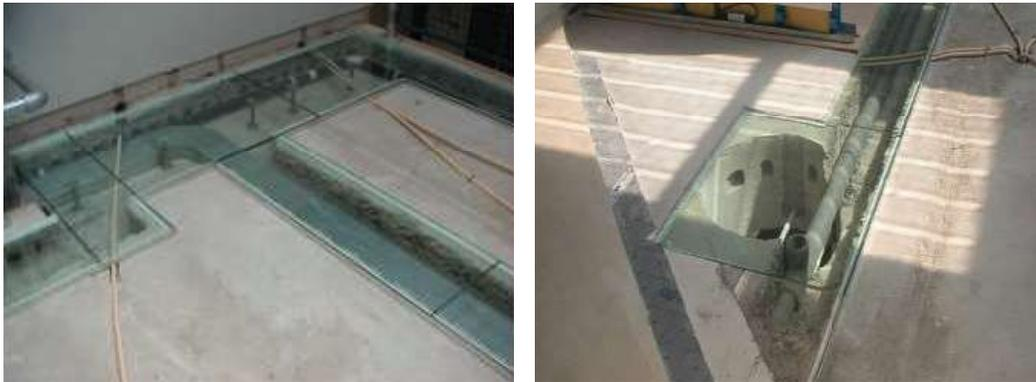
**Figure 25.** Hollow core units with ducts for pipes and conduits in the top flanges of the section makes "Pipe floor"
