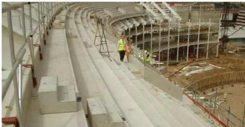
Figure 8. Precast terraces at Wembley Stadium using SCC, by Bison Concrete Products, 2007.
