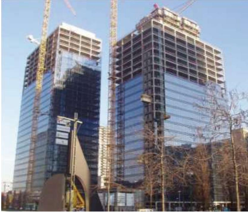
**Figure 4.** Precast tower block in Belgium, 36 storeys plus 6 storey basement, using high strength concrete in columns, shallow beams and lightweight floors. c. Egron, Belgium.
