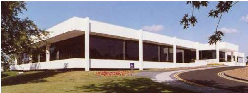
**Figure 9.** Polished precast concrete give a clean and white mock "marble" effects at a pharmaceutical's offices, Nottingham, UK. C. Trent Concrete Ltd., UK.
