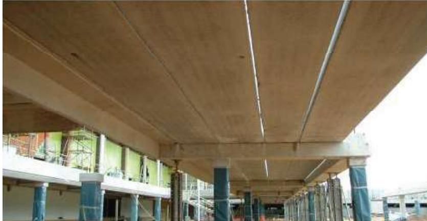
**Figure 11.** Prestressed concrete hollow core slabs spanning 16 m are 400 mm deep, and weigh just 5.2 kN/m<sup>2</sup>, 50% of a solid slab of the same depth.
